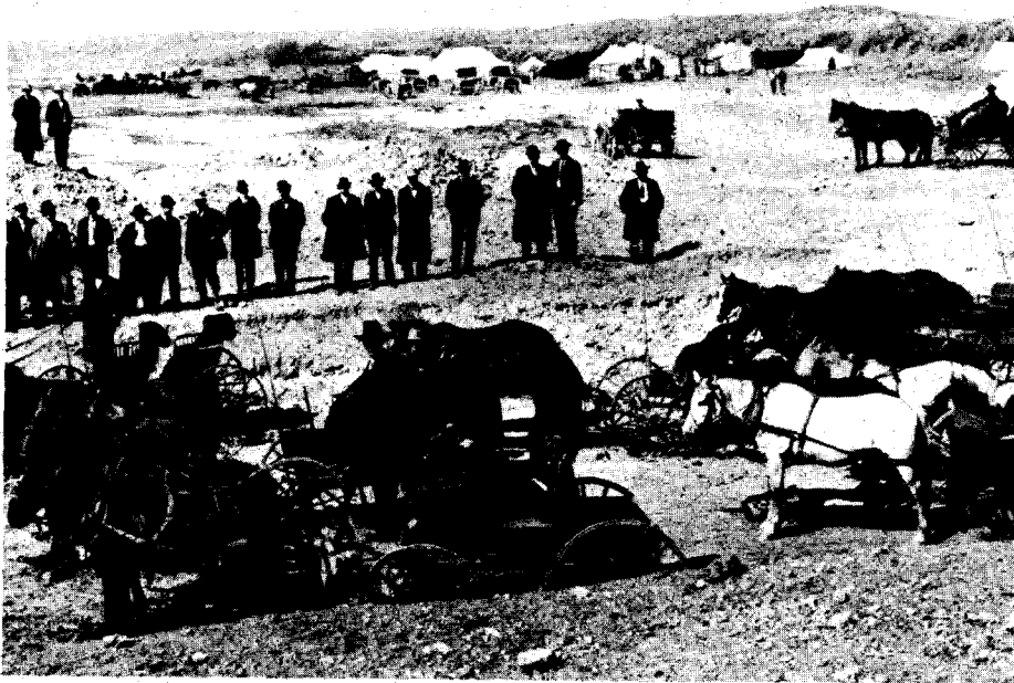
Construction of Lake Hattie Dam, circa 1909. Photographer unknown. From the Lewis Holliday Collection, courtesy of the American Heritage Center, University of Wyoming.
