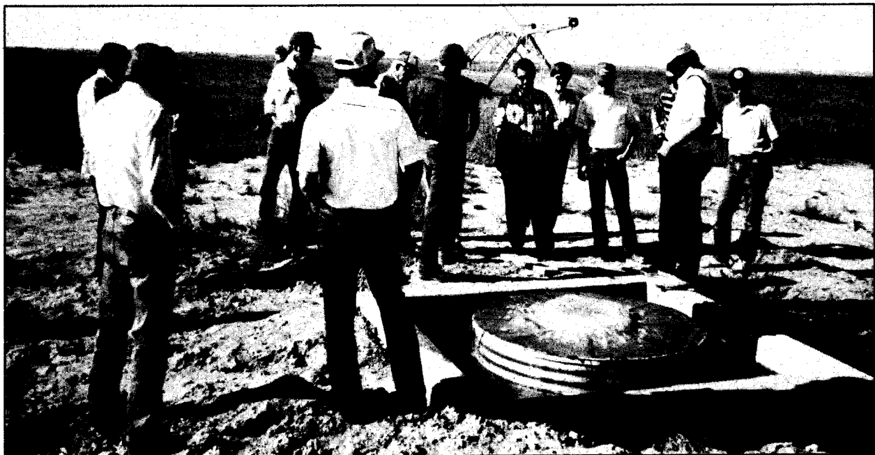
"Turbulent Fountain" type moss and vegetative trash screen for water used in a 95-acre, center pivot irrigation system on the Jim Hodder farm, Farson, WY. Canal water enters the base of the inner well via 10" PVC pipe with about 1.5-2.0 feet of head. The resulting fountain of water falls back into the well after passing through a screen rack.
