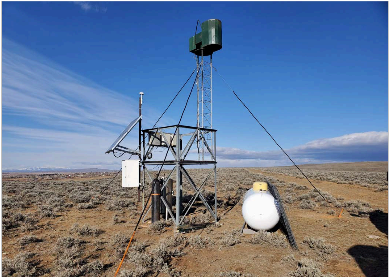
Figure 18. Looking SW at the Highland ground based generator site as it undergoes construction on 11 November 2021 Photo by WMI Technician Michael Paul.
