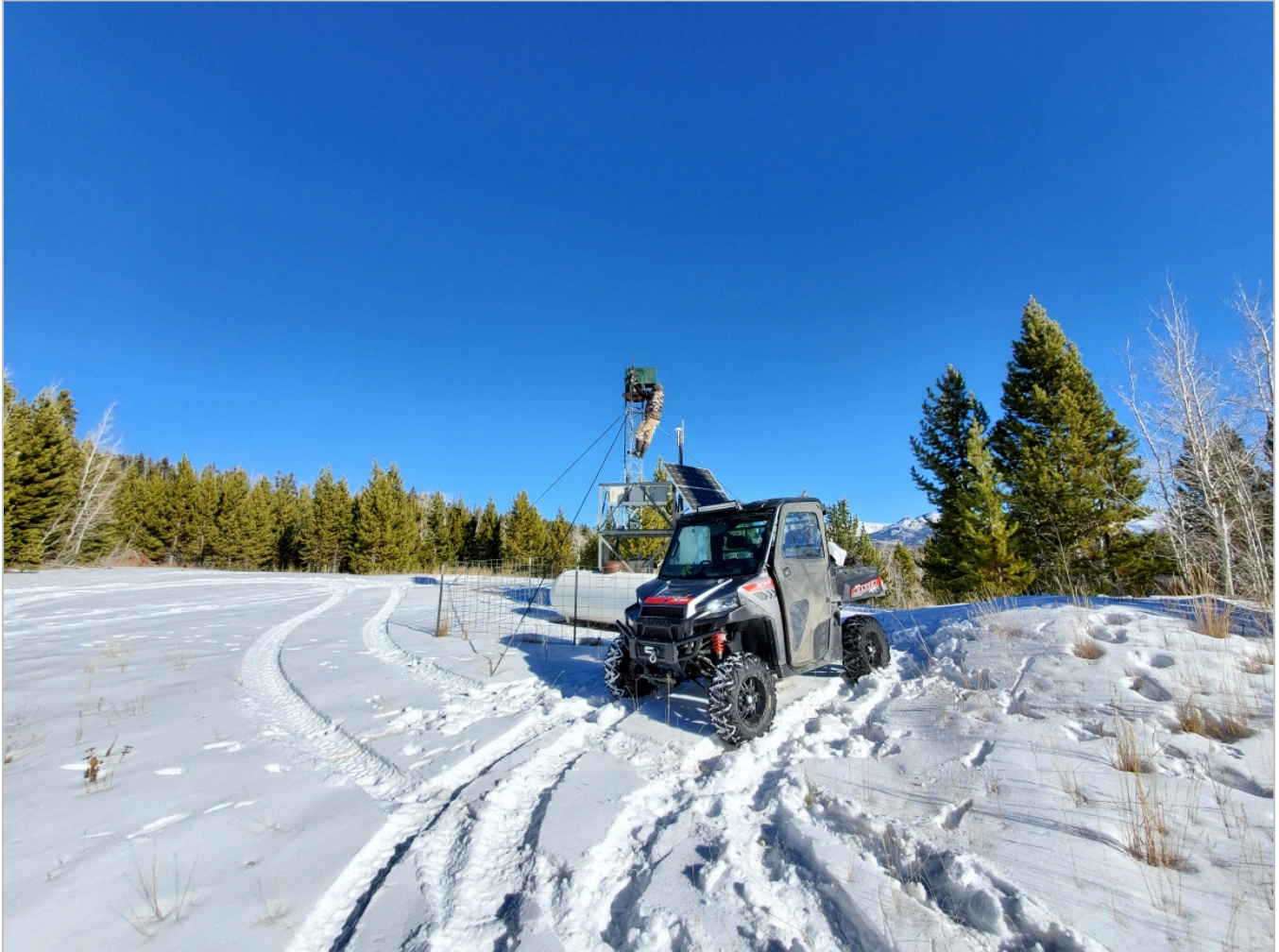
Figure 10. The WMI technician crew preform a maintenance check of generator WR01 (Big Sandy) on a clear day. Photo by WMI technician Michael Paul.
