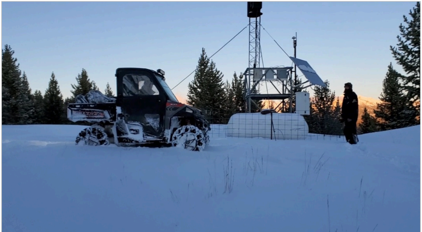
Figure 1. WMI Technicians finish up work on the ground-based cloud seeding generator at Big Sandy (WR01) as the sun begins to set. The crew was able to access the site this day via UTV. Photo by WMI Technician Michael Paul.
